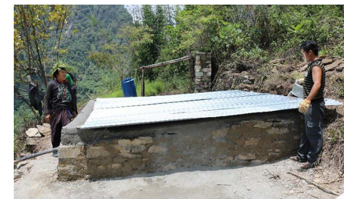
Soil Cement base Ferro Cement Tank at Yudrik Kengkhar Bhutan
